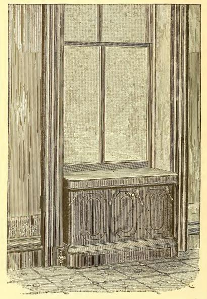
See plate III. description. The front view here shows the air-warming enclosure, with valves, and the projecting and overhanging top, from under which the warmed air is diffused downward into the room.
